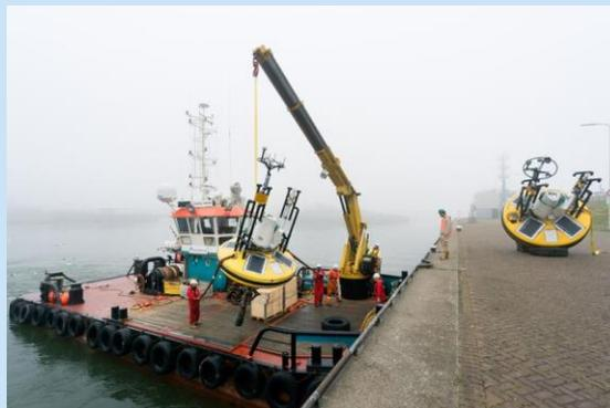
Source: Left: Installation of a met mast (Fugro Seacore); Right: Installation of a floating lidar device (RVO.nl).
